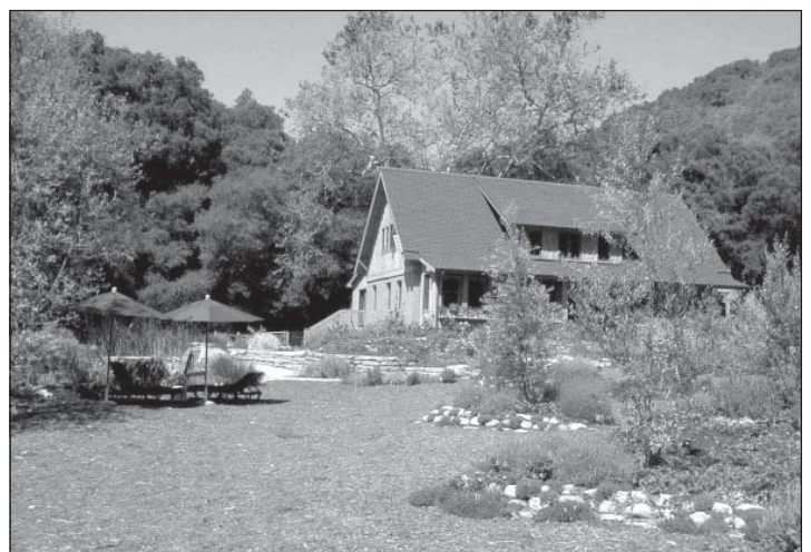
Straw bale house
